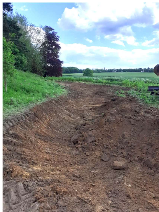
Completed works at Premier Foods
