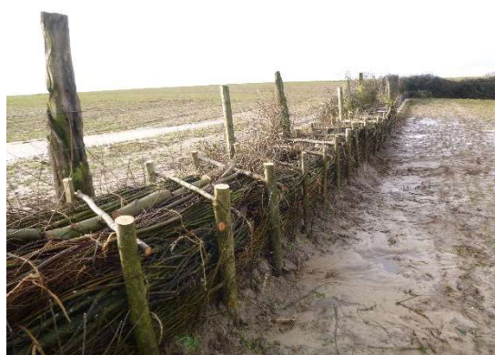
Newly created overland flow barrier (fascine)
